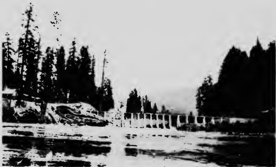
Canadian Collieries (Dunsmuir) Ltd. Storage Dam.
